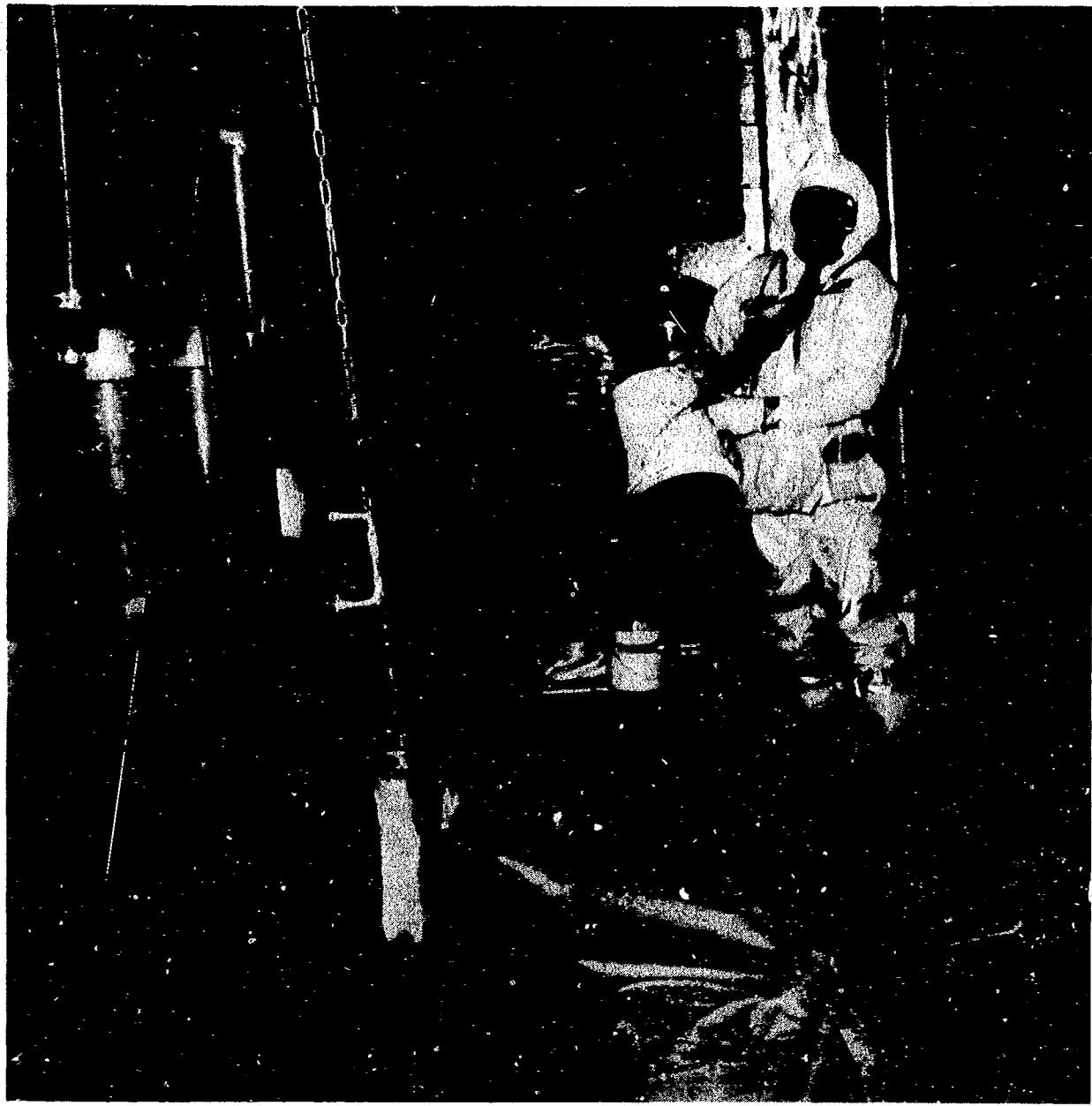
Figure 8. Sealant and a metal seal plate were placed between the refueling canal and the reactor vessel so the canal could have been flooded, if necessary, for shielding.
